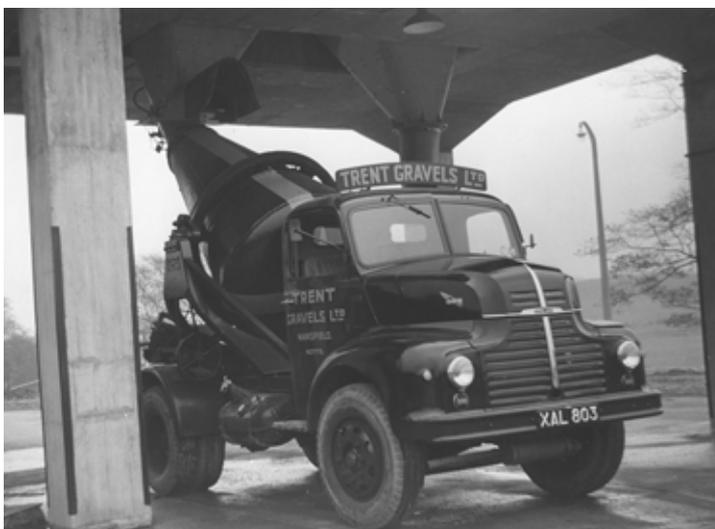
Loading an agitator at Trent Gravels' Mansfield plant
