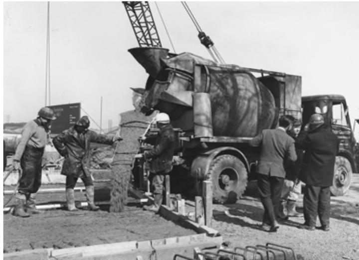
*A high-discharge truck working on the M1 in the early 1960s*
