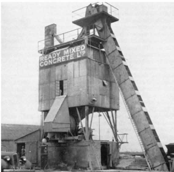
sand were handled by a bucket elevator and the plant had an output of up to 40yd<sup>3</sup>/h, which was discharged into six truck-mounted agitators, each capable of transporting 1½yd<sup>3</sup> of concrete. His vehicle fleet consisted of Chevrolets and subsequently included Studebakers.
