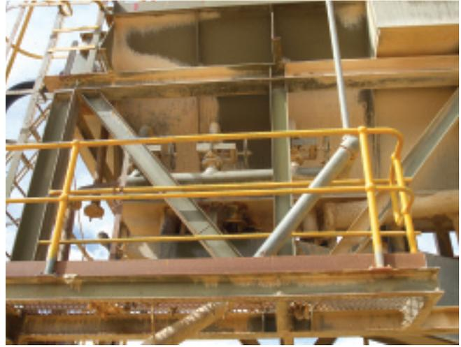
Fig. 3 External pipework for three RCCs
