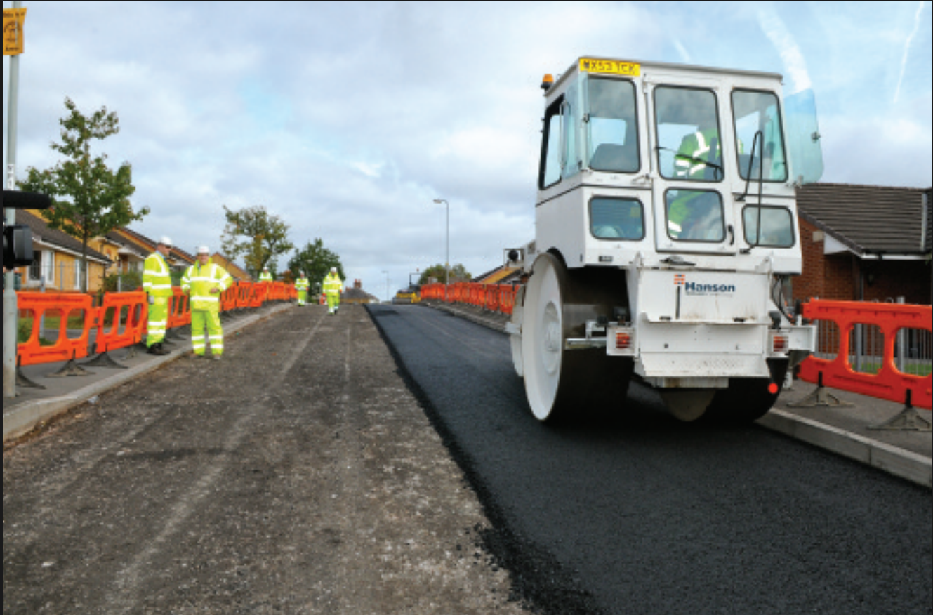
Hanson ERA (energy-reducing asphalt) reduces CO 2 emissions, enhances durability and improves health and safety for contractors
