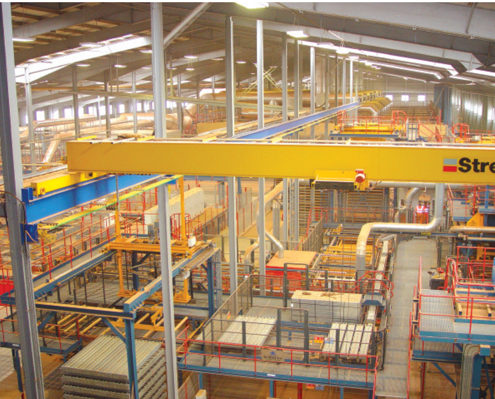
Part of Hanson Building Products' £50 million brick factory at Measham in Leicestershire
