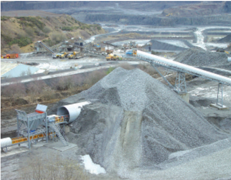
View of the new secondary surge pile with the old bottoming plant visible in the background
